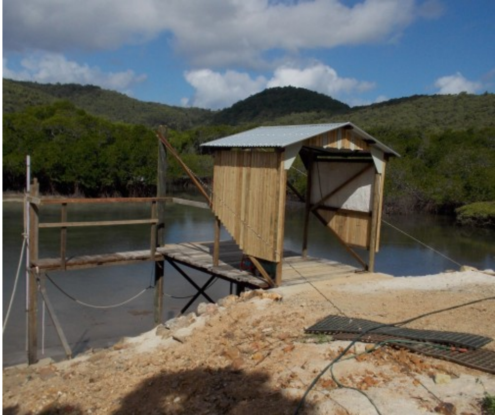
The new wharf in the lagoon
